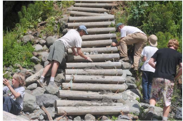
Volunteers repair the Houda Point beach trail (south side); Johnny Calkins, trail building and restoration expert, coordinated the effort.
