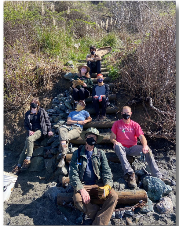
Ambassadors & volunteers proud of their work repairing the Baker Beach stairs.
