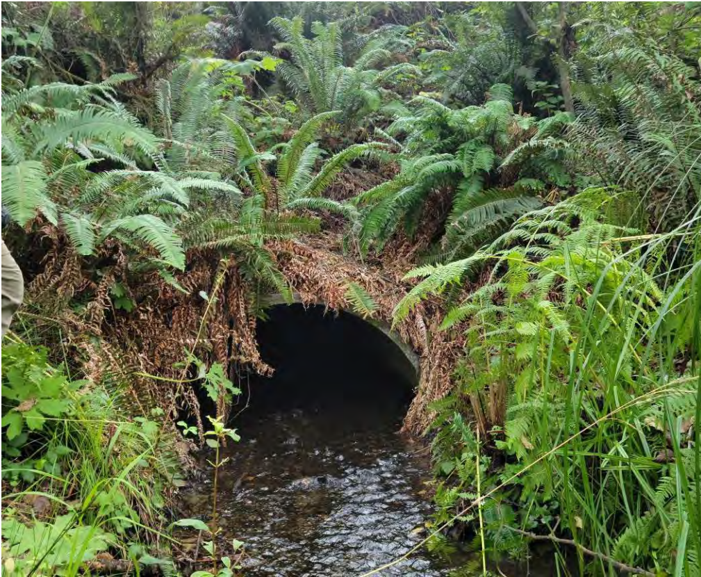
Photograph Location No. 7: Concrete culvert and flowing stream.
